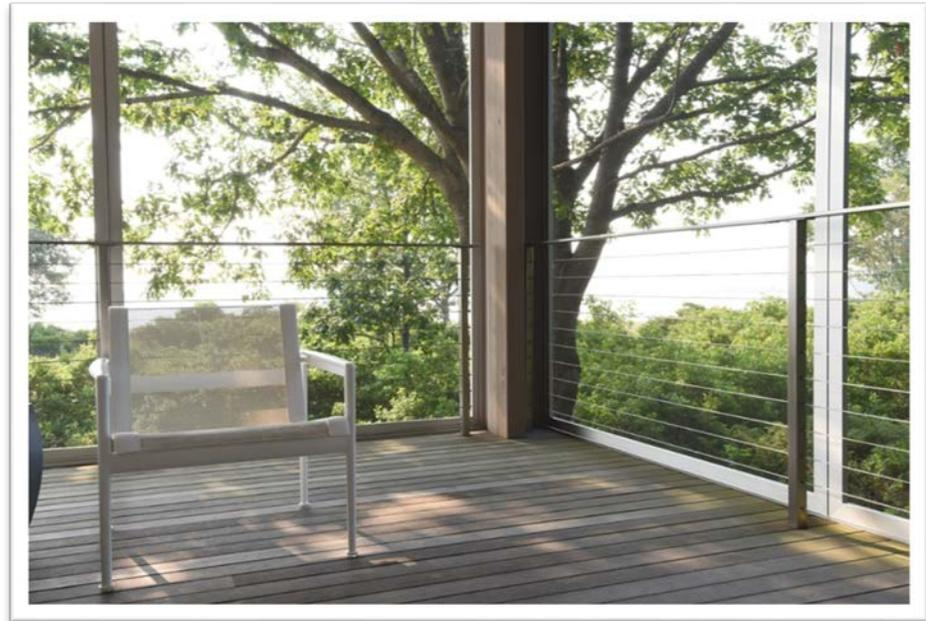
and tempered glass infill – for a fully-customized railing system at an affordable cost.
